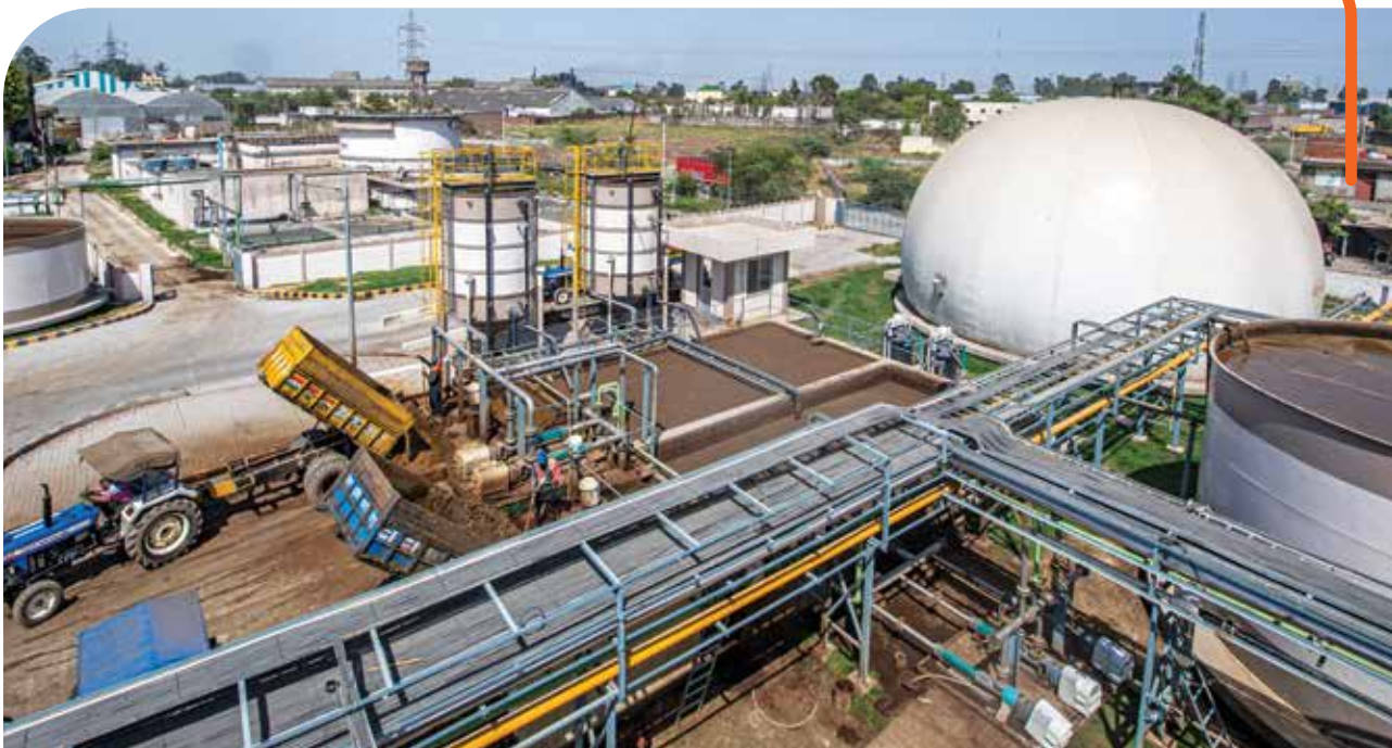
Recently established state-of-the-art biogas plant at Varanasi
